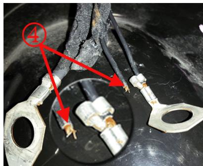
Technicians should inspect the ground for possible corrosion or damage at ground terminal ring, fasteners and grounding surfaces.
